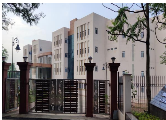
Diamond Jubilee Lecture Hall Complex National Institute of Technology Jamshedpur
